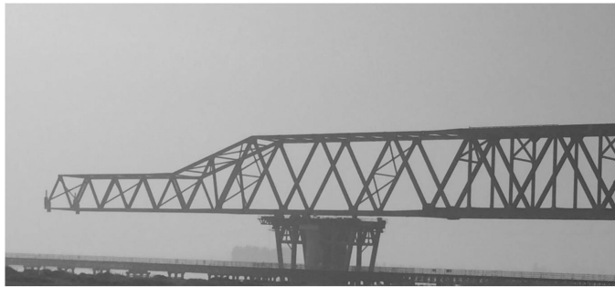
Fig. 4. The incremental launching truss bridge
